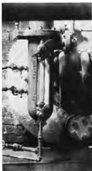
Fig. 1. Swivel Gage-Glass Guard.*
